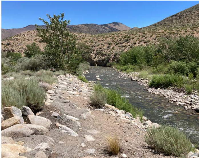
Modifications to river bank from 1997 post-flood repair to US 395
