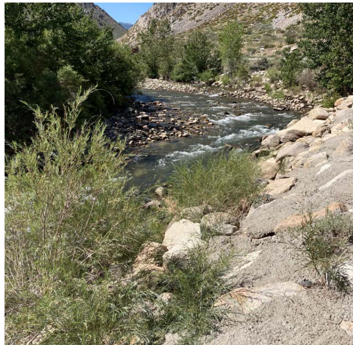
Modifications to river bank from 1997 post-flood repair to US 395
