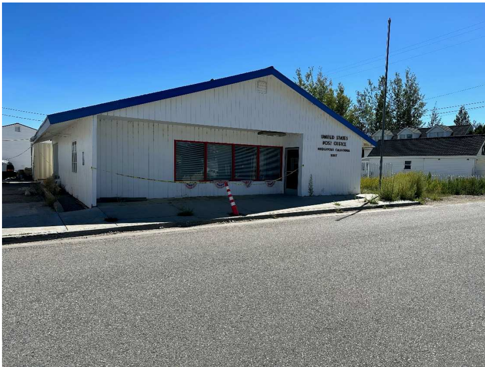
Bridgeport Post Office Building with caution tape.
